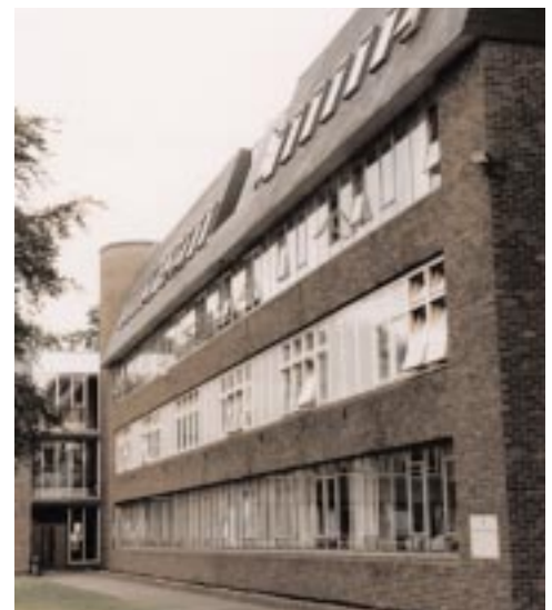
The refurbished building. The new window system on the first floor is the major component in the package of measures employed to avoid mechanical cooling
