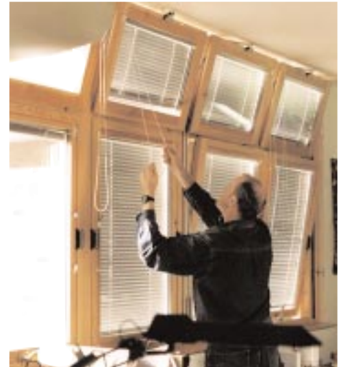
Figure 3 The upper and lower elements of the new windows are readily adjustable by the occupants
