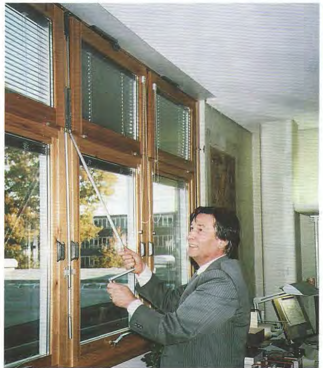
Figure 1 More usable controls can improve comfort and save energy. Effective control of windows and blinds helped to allow air conditioning to be avoided in this office refurbishment at the Open University. The upper windows, which permit secure night ventilation in the summer, are being adjusted
