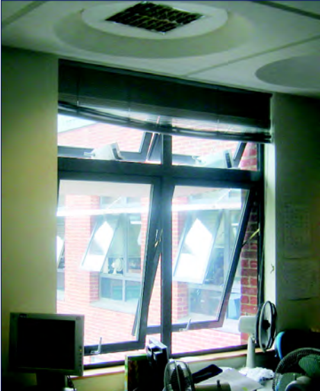
Above: Books were used to prop open fanlights that were never fitted with friction hinges.
