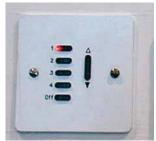
This control for lighting has clear switching with four settings clearly illuminated, plus an off setting. The numbers by the setting are arbitrary.
