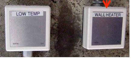
Over Summer 2009, this frost thermostat (improperly set at 17°C on installation) energised the wall heater in a plant room of a new low-energy school, and wasted more electricity than the wind generator (intended to offset the entire building's annual heating energy use) created.
