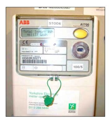
The principal sub-meter did not work, so the utility meter fault went five years undetected. The other sub-meters were wrongly calibrated, so cross checks were impossible.
