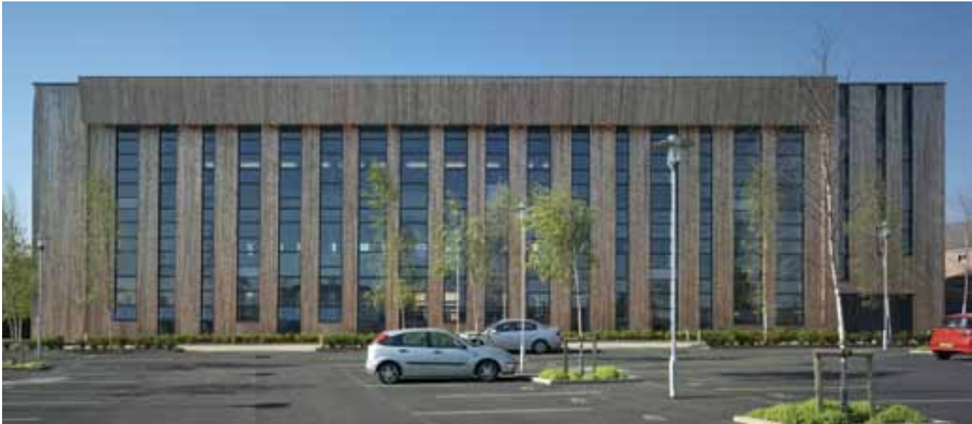
The Woodland Trust has a solid, cross-laminated timber structure, with external wood-fibre insulation and larch cladding
