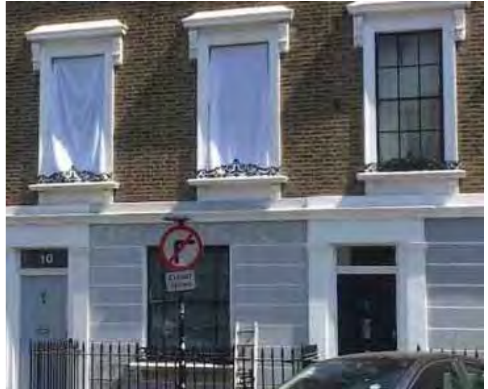
Ad hoc external shading by old linen sheets during 2022 London heatwave kept peak internal temperatures below 27 C.
