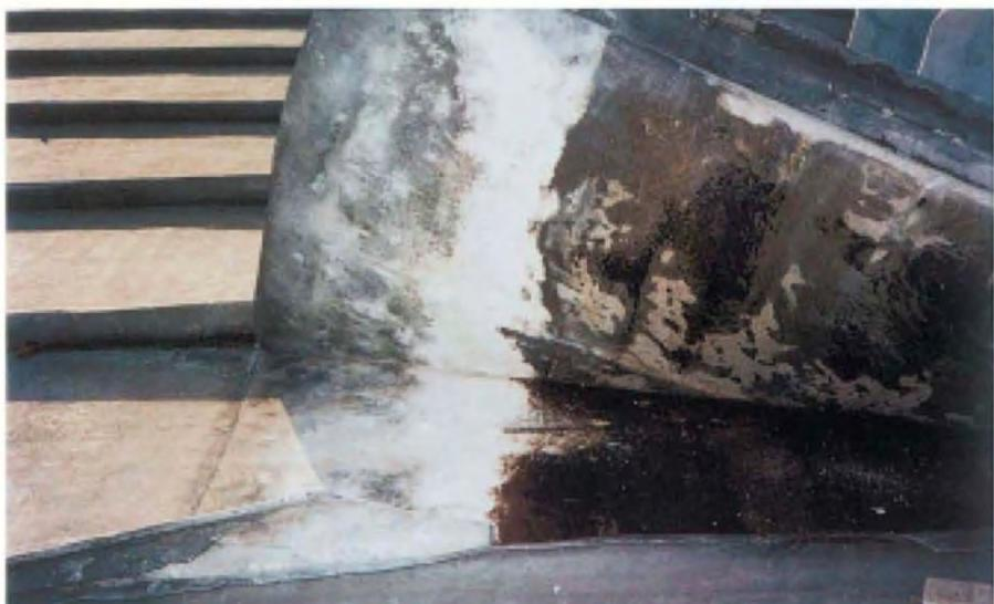
Figure 22 At this church in Yorkshire, roofing felt was used to protect the lead from acid vapours from the oak ceiling/decking. Although much of the lead has been protected, local membrane failure together with some water ingress has led to localised corrosion which in places has perforated the lead sheet.
