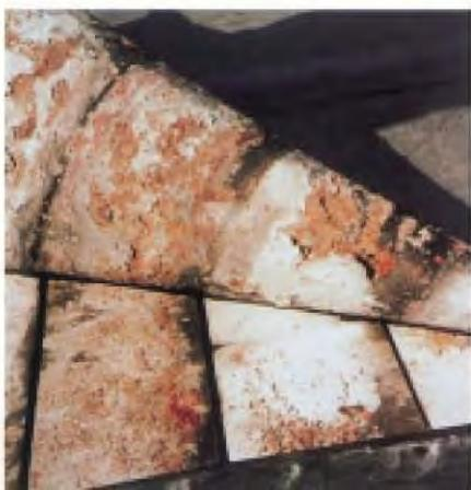
*Figure 15* *Village churches with oak ceilings which have lead laid directly above them are particularly susceptible to ULC. The reddish-brown coloration of lead oxide here is quite common, as are the passivated areas near the gaps where the acid vapours can disperse. In situations like this, where it is important to retain an oak ceiling, a Ventilated Warm Roof above may be the only answer.*
