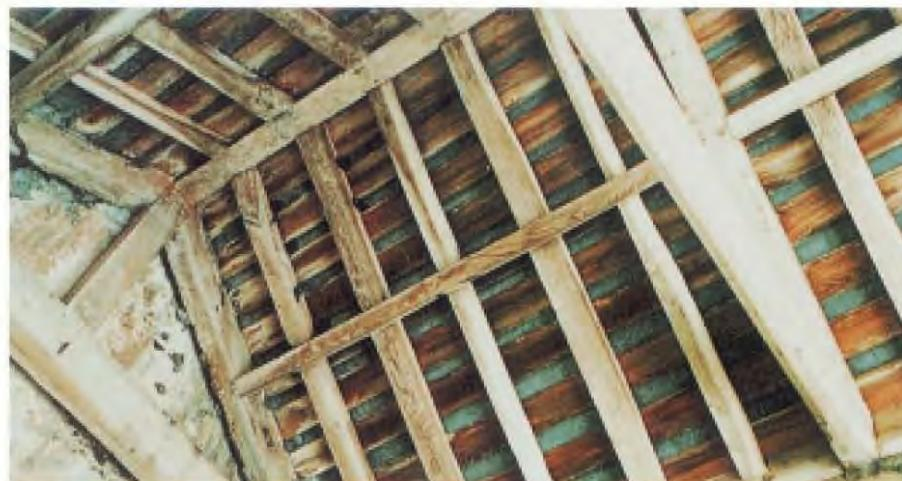
*Figure 20 A gap-boarded roof.* Softwood gap boarding is common in the steeply-pitched roofspaces of medieval cathedrals. It is normally unsuitable mechanically for flat or shallow-pitched roofs. For a variety of reasons, these roofs tend to be relatively resistant to ULC and the construction can often be maintained without any modification. A pretreatment on the underside can help to avoid initial corrosion. See Section 6.
