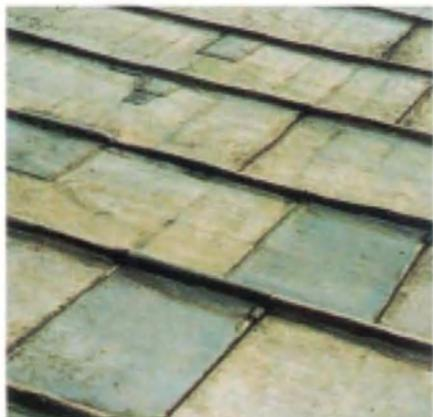
Figure 24 The large patches to the laps in the foreground suggest acid corrosion-related failures, which often first destroy the lead near the head of the lap. So do the smaller patches at the sides of the sheets, though similar damage can be caused by restrained thermal movement at tight fixing clips. The decking here is oak, probably 150–200 years old, but 35 years after re-leading, corrosion is severe.
