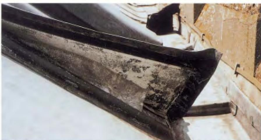
*Figure 16* *This early example of a VWR was ventilated from side to side, rather than from bottom to top. ULC has occurred in the less well-ventilated area near the eaves between the two bottom vents.*
