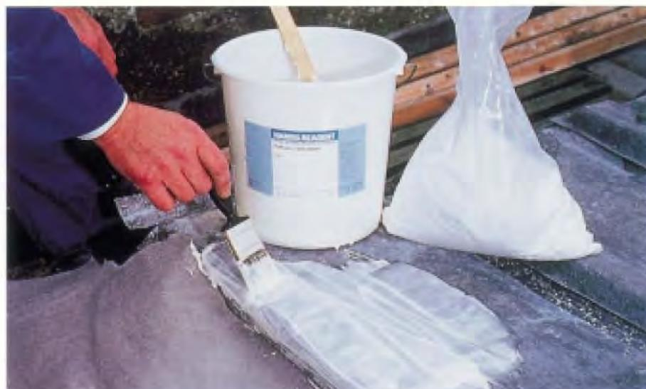
Figure 30 Applying the chalk slurry to the fresh lead. The coating thickness is sufficient when the surface of the lead can no longer be seen.
