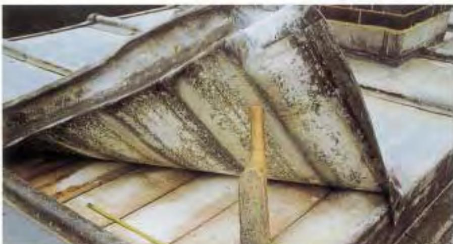
Figure 21 A typical corrosion pattern where lead has been laid directly over softwood boards in this historic house by the Thames, now used as offices. After 90 years, the underside of the lead is still in relatively good condition, but moisture and acids have caused some corrosion over the boards, while areas above the gaps are passivated. Note the heavier corrosion under the nosing, where trapped moisture is less readily able to disperse.
