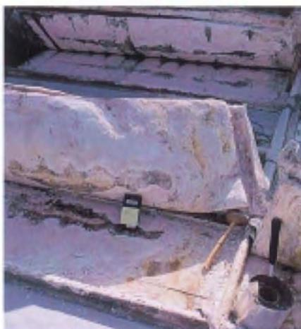
Figure 9 After forty years, ULC has consumed, on average, about one-quarter of the thickness of the lead here, and the roof is beginning to fail. Here, and frequently when ULC is severe, the prime cause is trapped moisture plus organic acids from the substrate: in this case hardboard over oak, which are both aggressive to lead. The rather less corroded stripes running up the sheets show where the rafters come.
