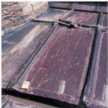
**Figure 2** This 1850s roof has eventually failed owing to fatigue cracks caused by thermal stresses in large sheets subject to constant thermal movement. A small amount of ULC was also visible under the sheets: this is perfectly normal, and has not contributed significantly to the failure.
