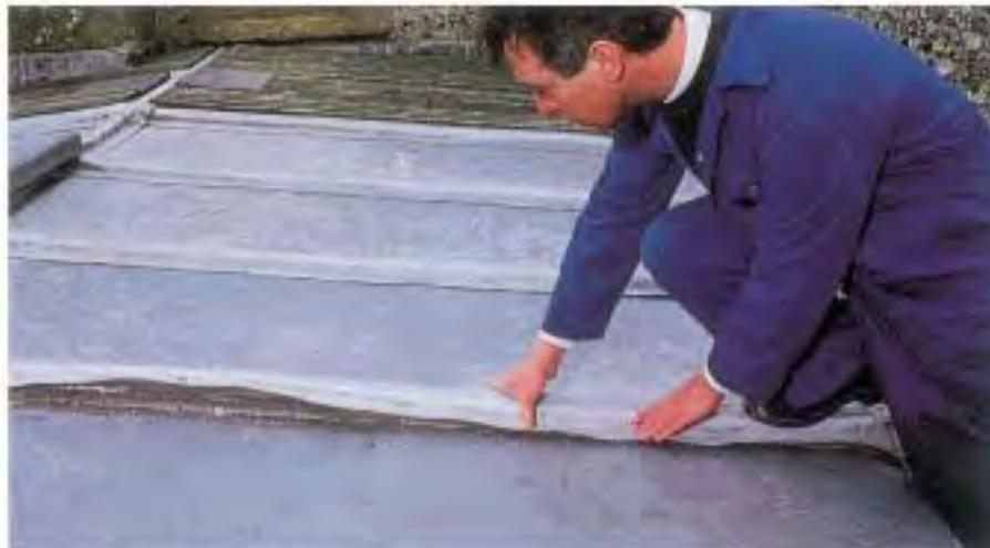
Figure 27 Replacing the lead
