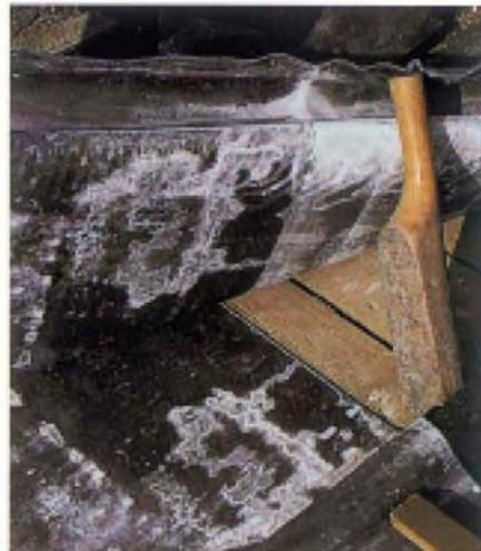
*Figure 18* In this VWR, the AVCL terminates some distance short of the abutment. The lead nearby has corroded underneath, which is to be expected in the circumstances. Some condensate has also entered the lap and caused local corrosion.
