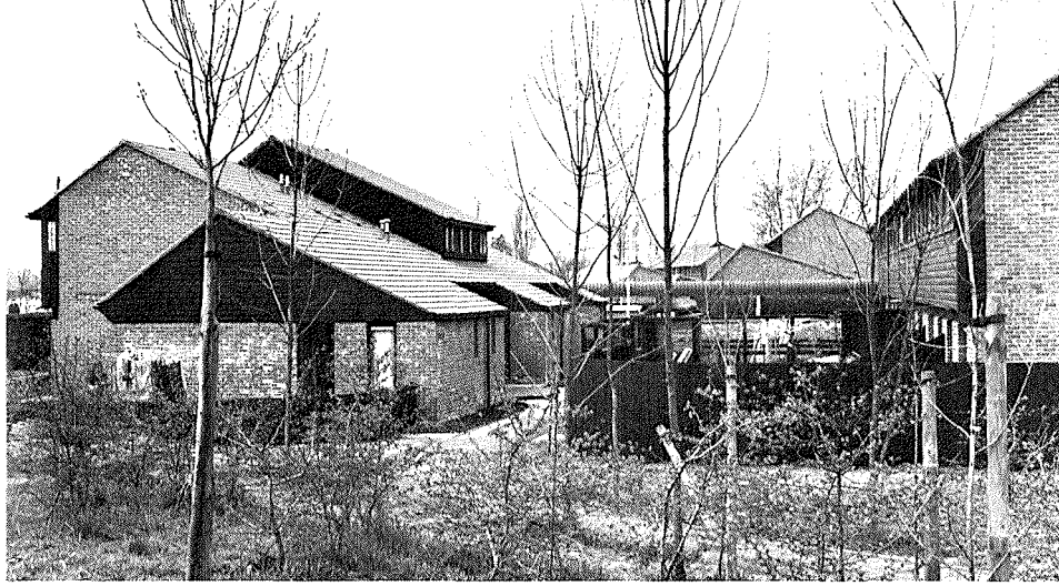
View of typical houses showing lower roofs at north side to allow sun penetration to the south side of the houses behind. High level duct with walkway under shows in the background.
