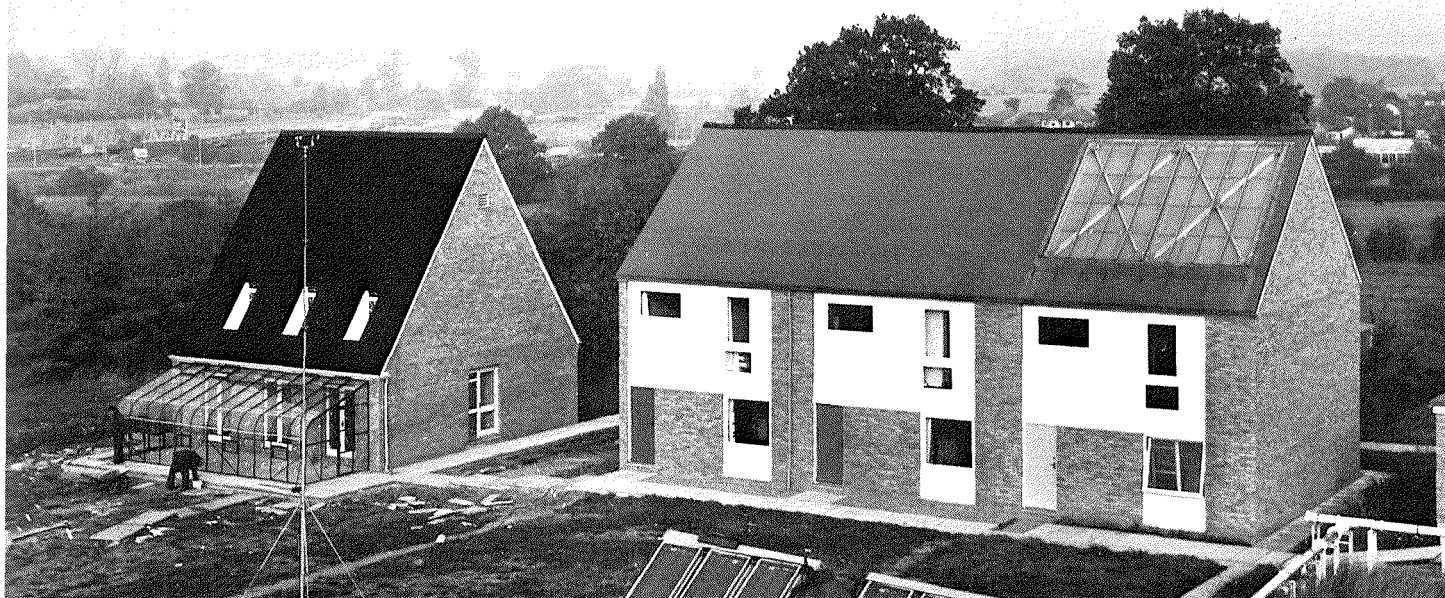
Heat Pump House at left, with terrace containing Heat Reclaim, Underfloor heating and Solar House at right.
