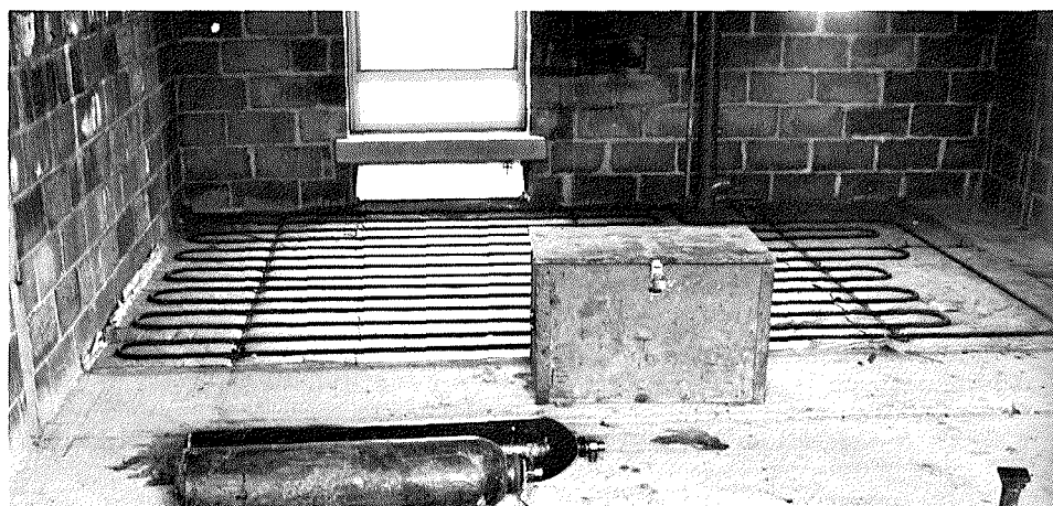
Steel floor heating coils from solar heating system
