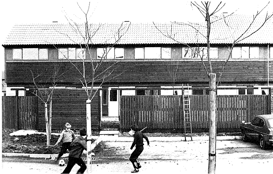
View of typical houses showing lower roofs at north side to allow sun penetration to the south side of the houses behind. High level duct with walkway under shows in the background.
