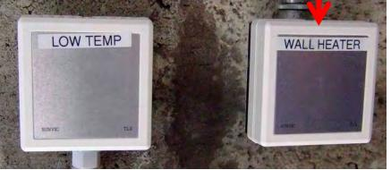
Over Summer 2009, this frost thermostat *(improperly set at 17° C on installation)* energised the wall heater in a plant room of a new low-energy school, and wasted more electricity than the wind generator *(intended to offset the entire building's annual heating energy use)* created.
