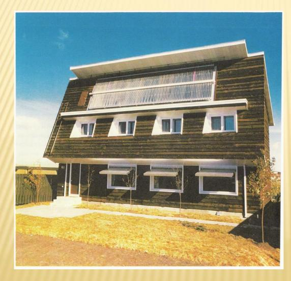
R-40 walls R-60 ceiling Triple-glazed windows Heat-recovery ventilation Drainwater heat exchanger 0.8 ac/h @ 50 pascals
