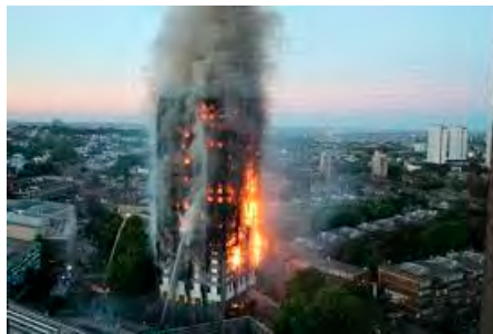
Figure 14. Grenfell Tower, London (Sources: https://en.wikipedia.org/wiki/Grenfell_Tower_ ).
