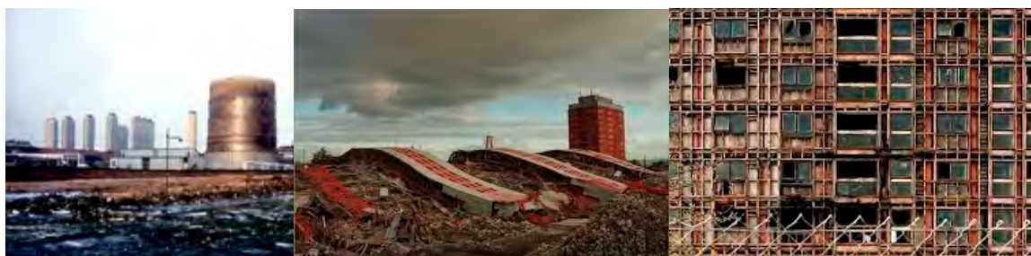
Figure 21. Red Road flats before and after showing the position of the asbestos sheeting.
