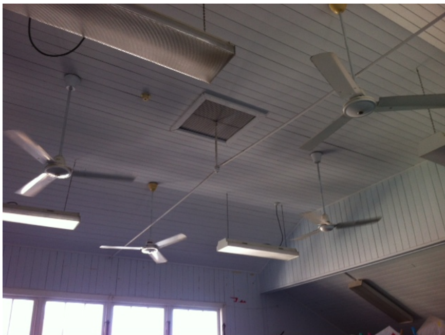
Figure 5.1 Ceiling Fans Mounted 4.1m from Floor & Centred in Classroom
