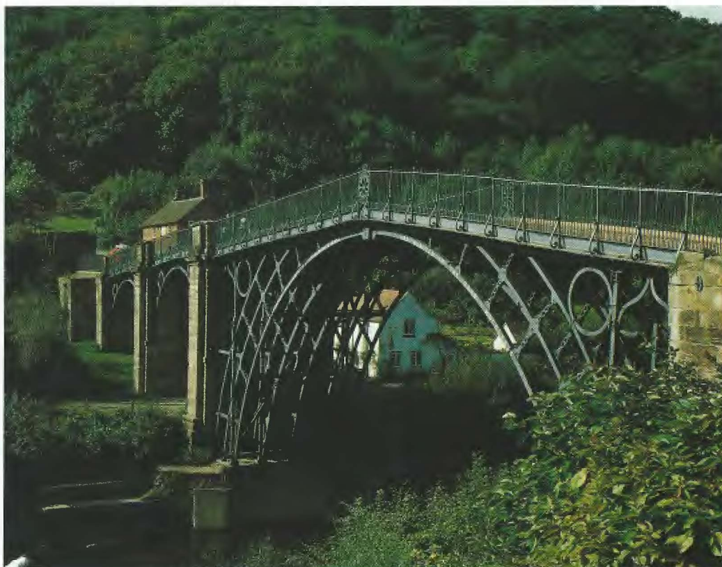
Plate 1. Abraham Darby's Iron Bridge at Coalbrookdale (1777–81) is a notable early example of the structural use of cast iron. From such precedents, cast iron warehouses, mills and factories were developed, many designed to be of fire proof construction.
