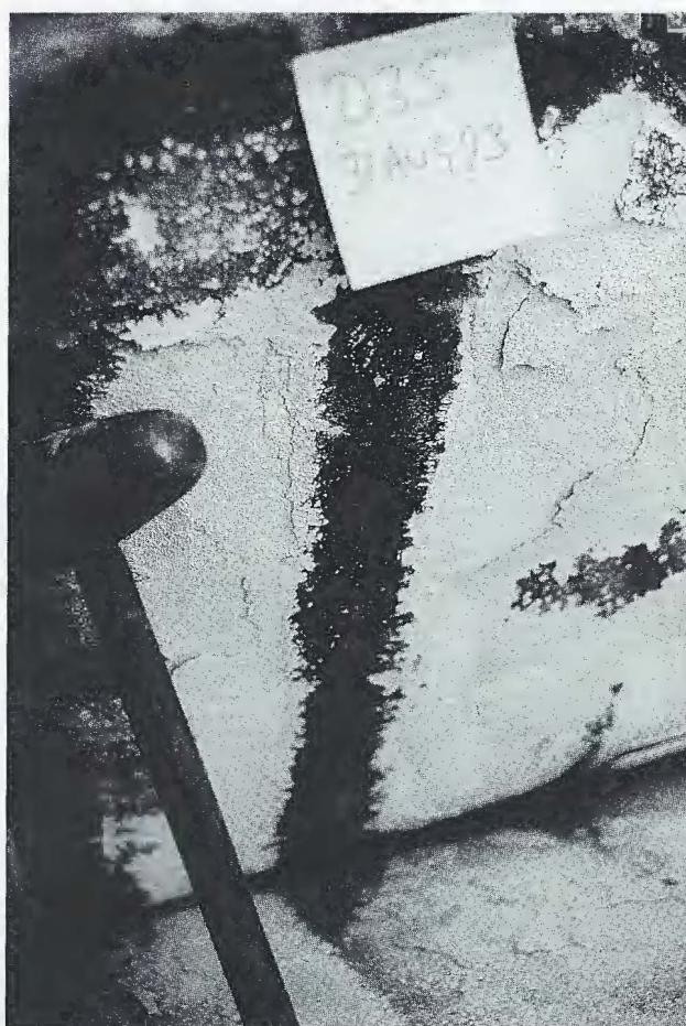
Figure 23. Passivated stripe at Donnington Castle. 3 mm hardboard separates the lead from the oak boarding underneath. The lead is badly corroded except for this dark passivated stripe, beneath which a softwood fillet was found under the hardboard. Since the acid content of the hardboard was found to be high (600 ppm) and similar throughout, the contrast is likely to be the consequence of different hygroscopic properties of the two woods.
