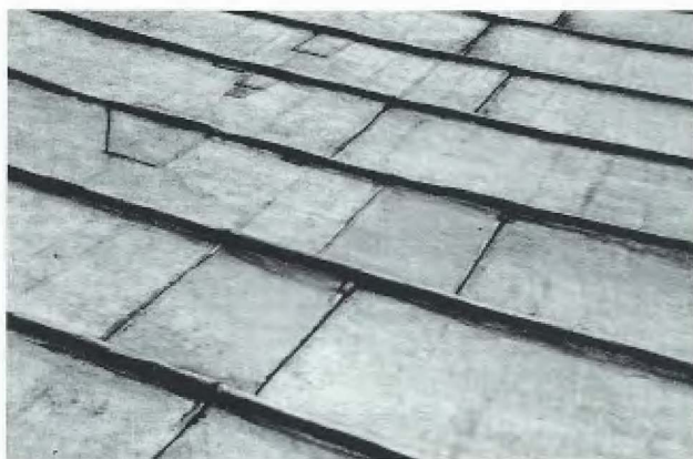
Figure 18. Norwich Cathedral cloisters, showing lead distress and repairs. The pattern here is characteristic of acid attack, with not only weakening along the gaps between the boards, but also failure at the perimeter, at rolls and laps. See also Colour Plate 9.
