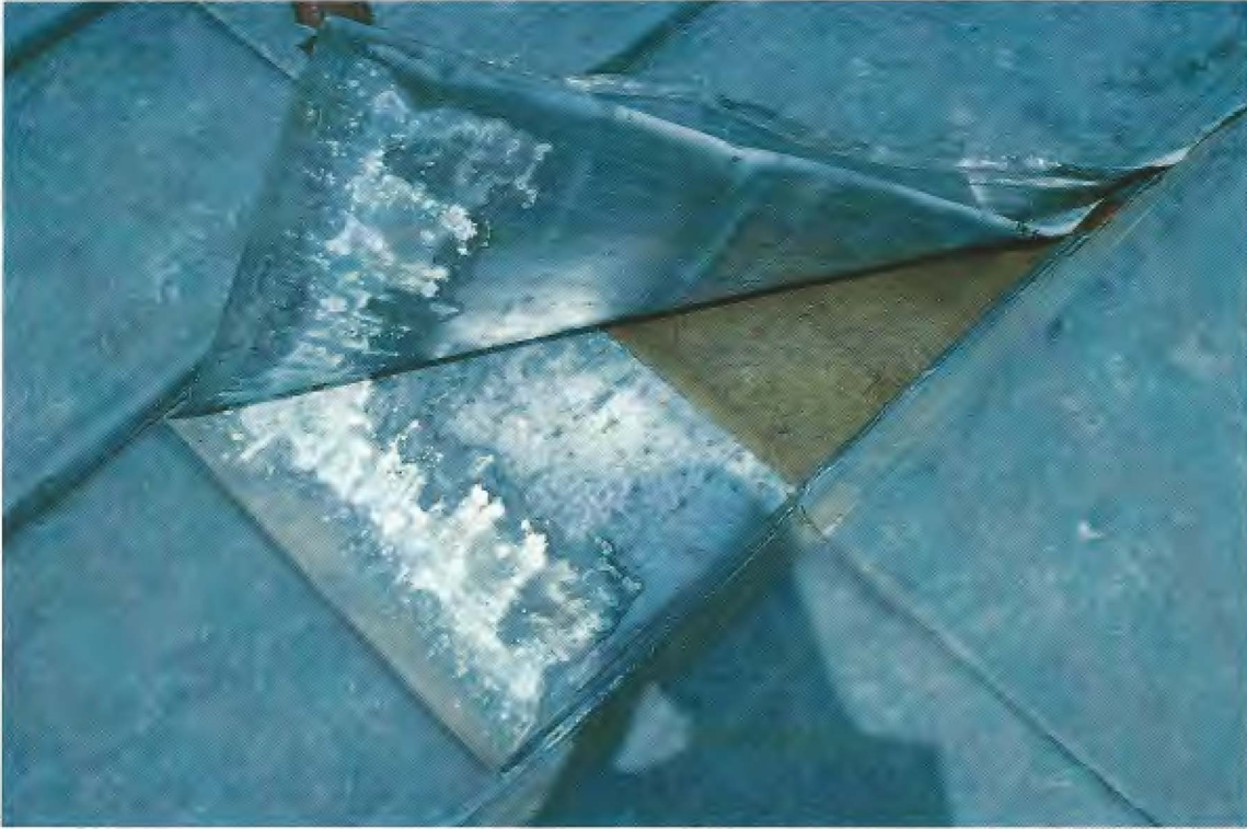
Plate 5. Lead over building paper on softwood on a relatively dry building. The lead is bright or only slightly dulled, though with a white haze between the boards. The pattern in the lap is not unusual: at the bottom a weathered area indicating capillary rise of rainwater, some corrosion (with a fringe of dark passivation) above that (where the rainwater distils) and the lead above that unaffected. The hollow rolls are free from corrosion. See also Figure 11, p 41.
