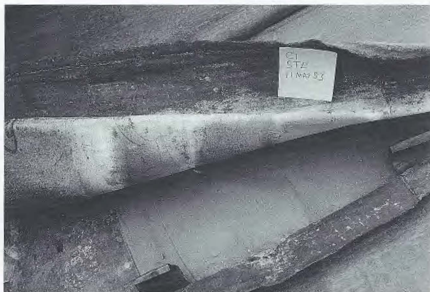
Figure 14. Corrosion over geotextile in a ventilated warm roof. While not serious, the underside lead corrosion is considerably greater than where the lead is placed directly on low-acidity softwood boards in ventilated warm roofs which are properly vapour-sealed from the building below.
