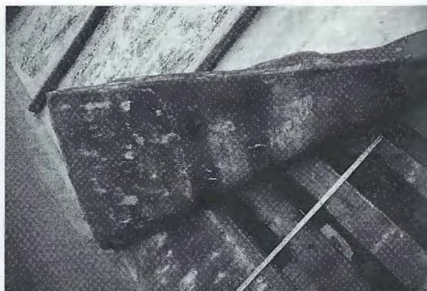
Figure 9. Lead over gap-boards at the Church of St Cross, Winchester. This lead, which dates from the 1880s, is generally passivated above the gaps and very slightly corroded over the boards. As in Figure 8, there has also been some slippage. To get some corrosion in the lap is not uncommon.
