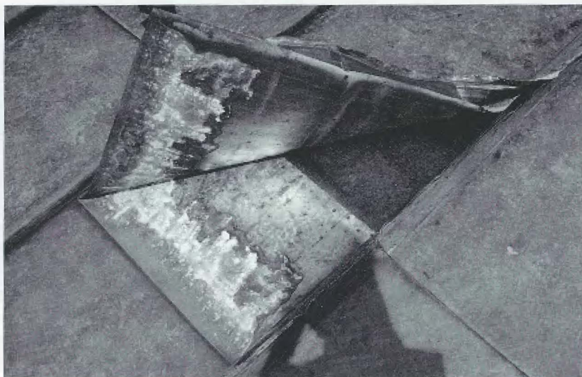
Figure 11. Lead over building paper on softwood on a relatively dry building. The lead is bright or only slightly dulled, though with a white haze between the boards. The pattern in the lap is not unusual: at the bottom a weathered area indicating capillary rise of rainwater, some corrosion (with a fringe of dark passivation) above that (where the rainwater distils) and the lead above that unaffected. The hollow rolls are free from corrosion. See also Colour Plate 5.
