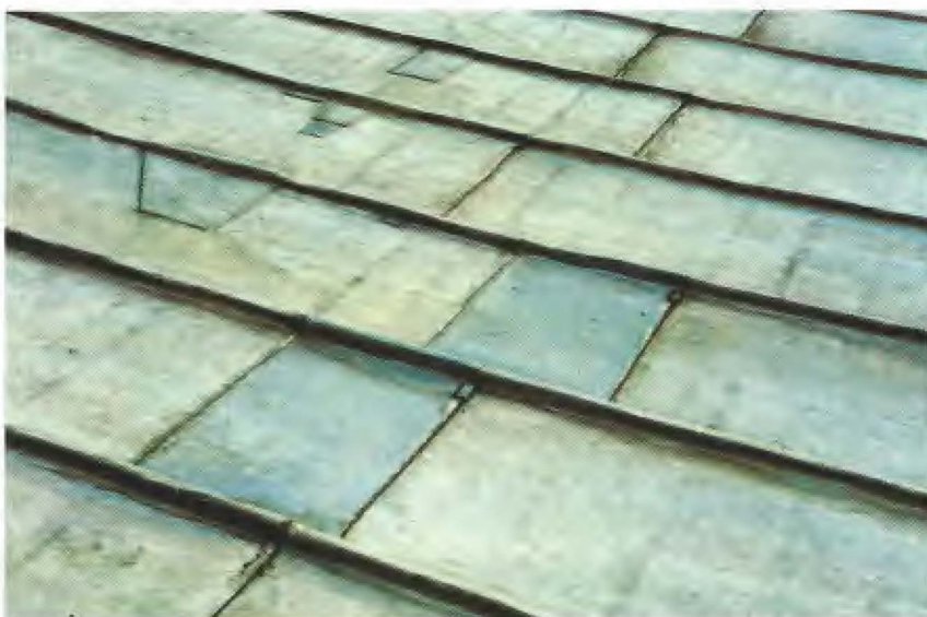
Plate 9. Norwich Cathedral cloisters, showing lead distress and repairs. The pattern here is characteristic of acid attack, with not only weakening along the gaps between the boards, but also failure at the perimeter, at rolls and laps. See also Figure 18, p 44.
