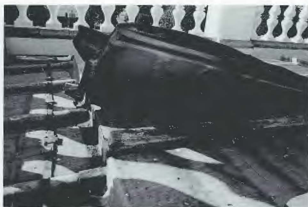
Figure 13. Underside of lead over Erskine's felt in a damper location at the Dorset mansion. The lead above the gaps is somewhat corroded, particularly towards the rolls in which there is also some corrosion. Note also the corrosion in the rolls above the splashlaps, as in Figure 12. The splashlap corrosion pattern varies with the distance apart of the sheets. Water is also trapped in the splashlap here by a slight backfall below the nosing. See also Colour Plate 7.
