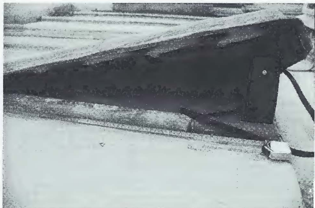
Figure 15. Rapid initial corrosion at a mansion in Buckinghamshire. Four weeks after this sheet was replaced in the autumn, fish-tails were already very evident.
