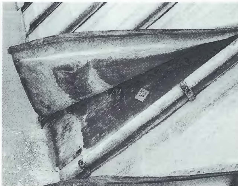
Figure 24. The south-facing roof of the Great Hall at Hampton Court. Corrosion is greatest around the perimeter and in places where the lead has bulged away from the substrate. The corrosion in the rolls varies from place to place and from sheet to sheet, presumably depending upon the precise geometry and its propensity to trap moisture.
