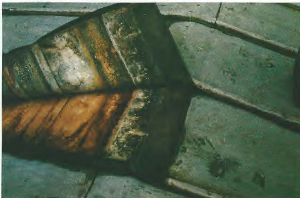
Plate 2. Corrosion above softwood boarding. White and yellowish (States 1 and 2) corrosion product on the nave roof of a Buckinghamshire church, with dark passivation above the gaps between the boards. The photograph was taken after a cold, clear night, and the roof was particularly damp at the time. Note also the passivation over the rolls (with the odd spot of corrosion). The ridge is passivated on the far (right) side, probably by rainwater, which also seems to flow over the ridge from time to time (the lap is mean). Not surprisingly, there are signs of corrosion here, probably the result of a combination of condensation and refluxing of rainwater. In spite of this, and of the church being particularly damp (RTL 1993, Report 6, Appendix D), the corrosion is not yet serious. See also Figure 6, p 38.
