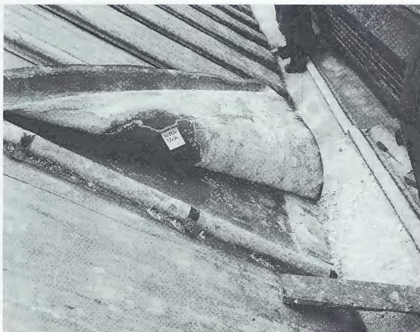
Figure 25. The north-facing roof of the Great Hall at Hampton Court. While this sheet generally exhibited more corrosion, it has a highly passivated area in the middle. Contrasts like this also occur on the south side.
