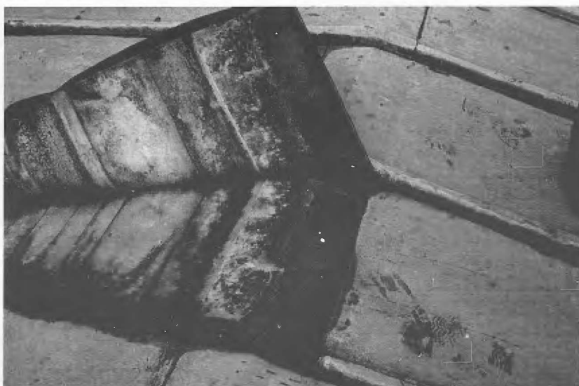
Figure 6. Corrosion above softwood boarding. White and yellowish (States 1 and 2) corrosion product on the nave roof of a Buckinghamshire church, with dark passivation above the gaps between the boards. The photograph was taken after a cold, clear night, and the roof was particularly damp at the time. Note also the passivation over the rolls (with the odd spot of corrosion). The ridge is passivated on the far (right) side, probably by rainwater, which also seems to flow over the ridge from time to time (the lap is mean). Not surprisingly, there are signs of corrosion here, probably the result of a combination of condensation and refluxing of rainwater. In spite of this, and of the church being particularly damp (RTL 1993, Report 6, Appendix D), the corrosion is not yet serious. See also Colour Plate 2.
