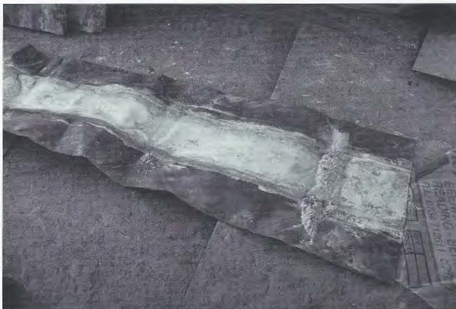
Figure 28. Lead over plywood in a gutter, with woodwool slabs to each side.
