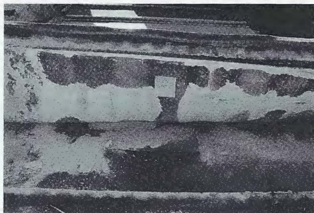
Figure 22. Typical underside corrosion patterns at Donnington Castle. A rafter underneath in the foreground coincides with the less-corroded area at the top.
