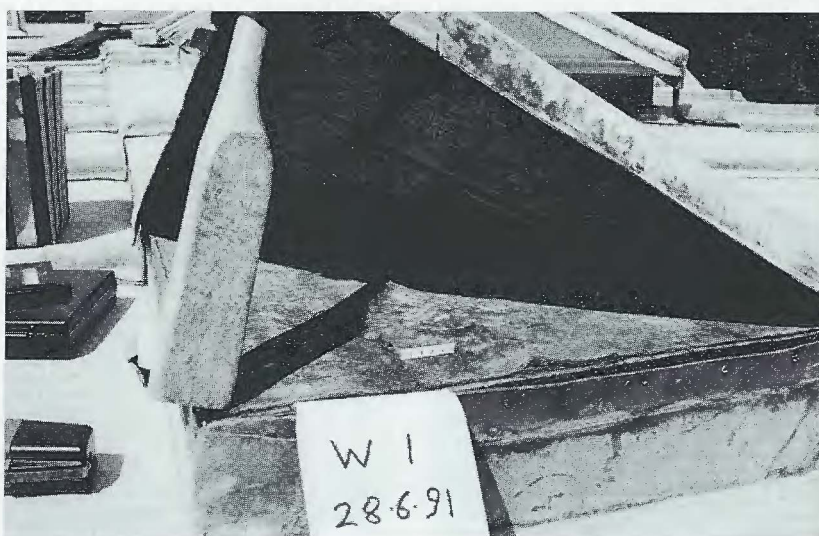
Figure 17. The original roof at the mansion in Buckinghamshire. Most of the roof was laid over Erskine's felt and was passivated between and corroded above the boards (the opposite of the current pattern). A few sheets, which did not have the felt, showed a similar pattern but with worse corrosion over the boards, probably because any moisture accumulating within this region would be trapped for longer than over the more permeable felt, and possibly there might have been some acidity. The longitudinal stripe was made by wire-brushing for tests and is not part of the original pattern. See also Colour Plate 8.
