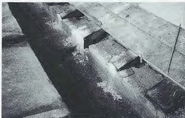
Figure 21. Valley gutter at the church near Sheffield. The lead from the gutter and roof has been removed in preparation for replacement by a ventilated warm roof. Products of corrosion at the oak rafter ends are very evident.
