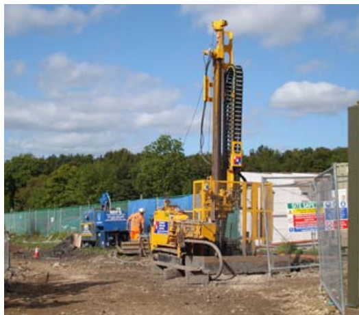
Borehole drilling for Bramall Learning Centre at RHS Garden Harlow Carr
