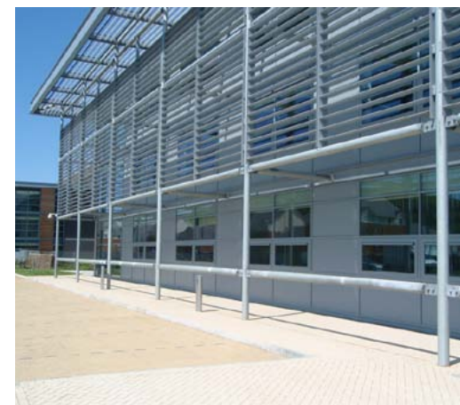
Ceredigion County Council brise soleil on south facade
