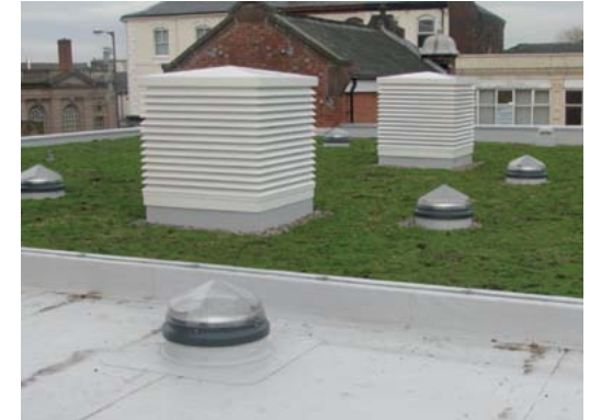
Wind catchers at Stoke Local Service Centre overcome the issue of a deep floorplate
