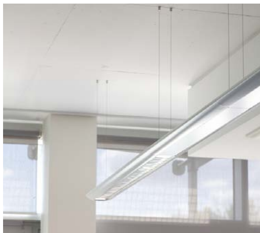
Thermal mass in exposed concrete slab at City Academy, Hackney
