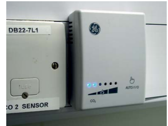
A 'traffic light' display at City Academy shows air quality in the room and indicates when the windows should be opened
