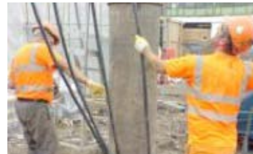
Installing a ground loop for a ground source heat pump system
