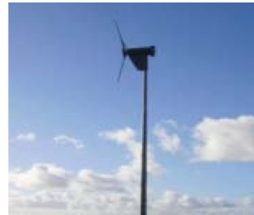
Installed 6kW wind turbine at Breezydaze, Cornwall
