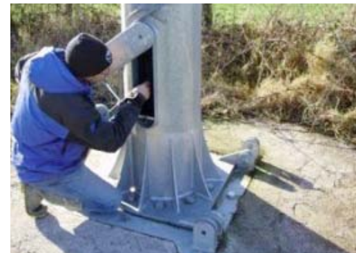
Access to manual brake on Breezydaze wind turbine
