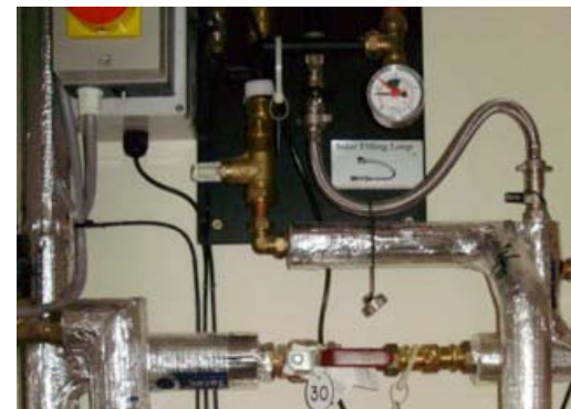
Example of labelling for maintenance on Trafalgar Nominees' solar thermal system
