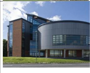
West Suffolk House: a naturally-ventilated office in Bury St Edmunds, with an open loop ground source heat pump, and solar thermal hot water heating.
