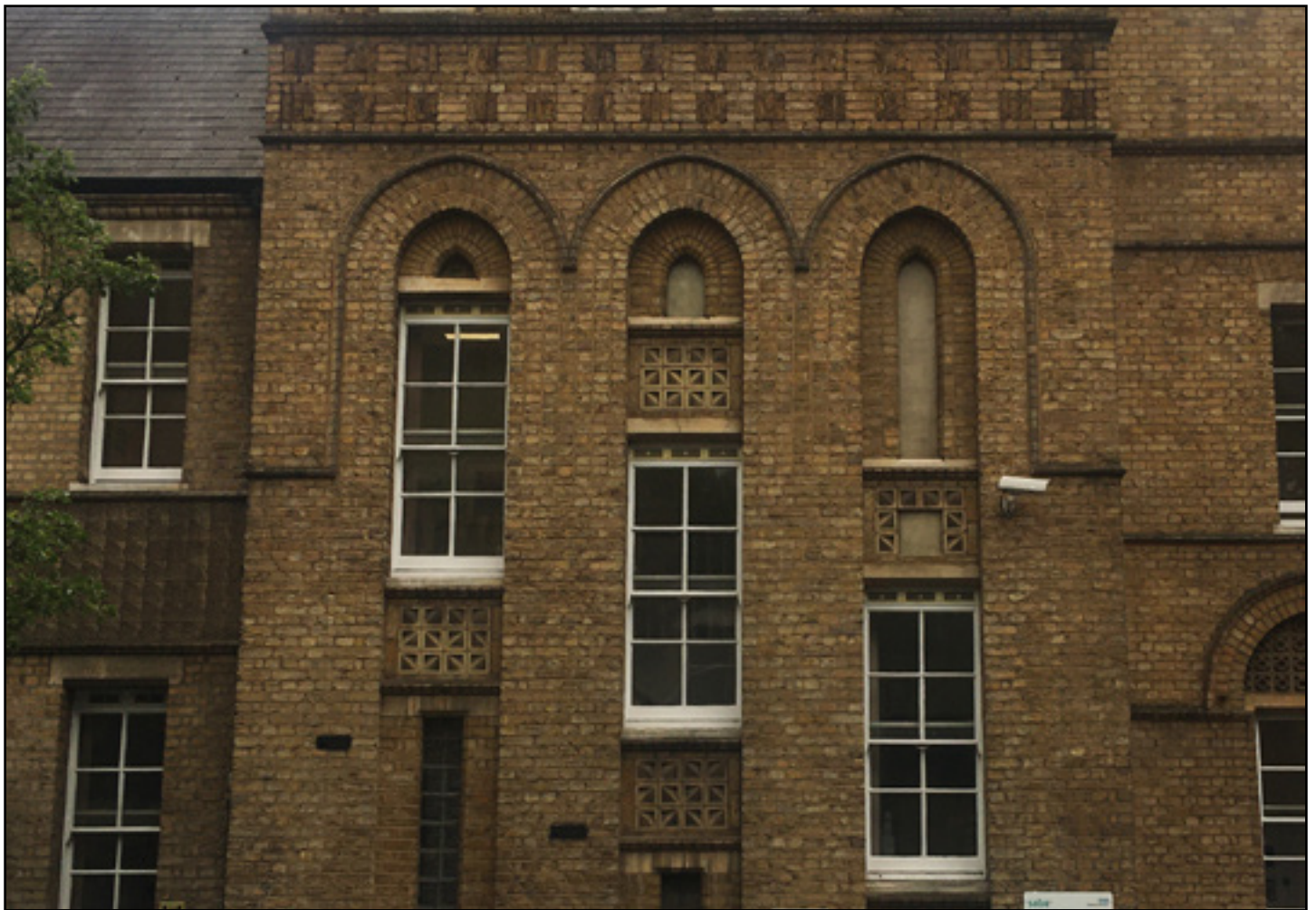
Figure 9. Traditional buildings were designed to function without operation energy input: staircases, for example, were provided with windows. (Photo: Robyn Pender).
