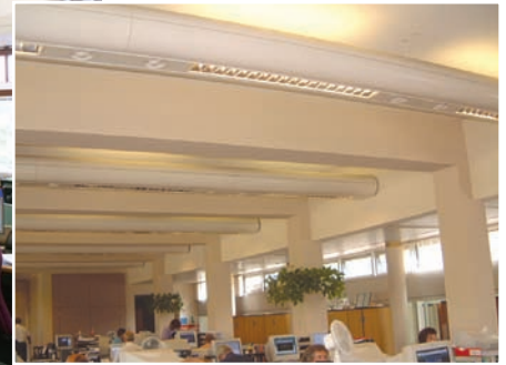
LEFT: The introduction of flush floor trunking runs have freed up the layout in the refurbished offices ABOVE: Uplighters, providing only patchy lighting in the building before its refurbishment, were the basis of one of the occupants' complaints
