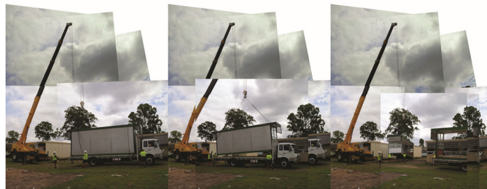
Figure 4: Deployment of a Mk I demountable classroom module.
