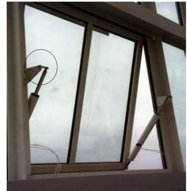
*The occupier has had to add new brackets and fixing plates. The same actuators fixed to the lower mullion would reduce the forces acting on each actuator and simplify the fixing, but would be more visually intrusive.*
