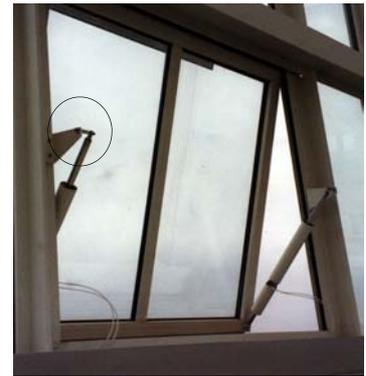
*The occupier has had to add new brackets and fixing plates. The same actuators fixed to the lower mullion would reduce the forces acting on each actuator and simplify the fixing, but would be more visually intrusive.*
