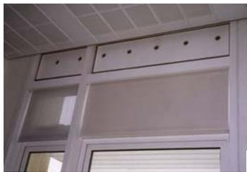
This office building in Northampton used fixed trickle ventilators and natural ventilation to maintain IAQ, plus a mechanical system (supplemented by chilled beams) for summer cooling. In practice the amount of trickle ventilation has proved excessive, and sometimes draughty; and many of these ventilators have now been blocked-up. However, in other respects natural ventilation via the atrium is working well. High level atrium vents are operated by paired pneumatic actuators. See Reference [9.]
