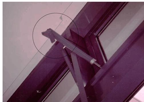
*The pneumatic linear actuators operating these motorised fanlights at the top of an atrium are virtually in the plane of the window when closed, leading to large turning moments and shear forces, also applied eccentrically to projecting studs from the brackets. After four years, this had proved too much for the self-tapping screws fixing the brackets to the mullions. The occupier has had to upgrade the fixings with bolted connections.*
