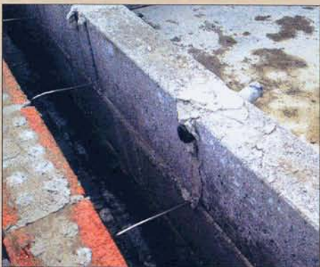
Underslab insulation in line with Perinsul block for continuous insulation (left); stainless steel cavity wall ties and inbuilt hoses for injecting full fill insulation (centre); and 200 mm cavity closers (right) are fitted to all openings in the cavity
