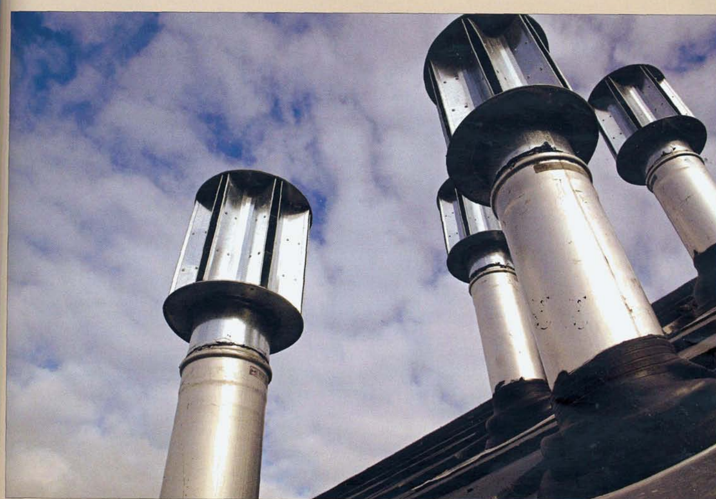
The passive stacks originate (below) in each of the wet rooms in the dwelling and rise vertically through the building and terminate above the roof (above)
