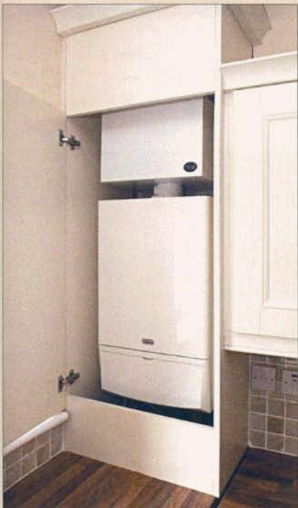
The Zenex Gas Saver (above) sits on top of the Alpha condensing gas boiler, bringing the boiler efficiency up to 98% by using a passive flue heat recovery device to recover heat from the flue gases of the boiler more efficiently than the boiler does
