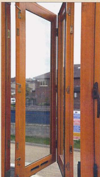
The supply air windows (above) open here to reveal their innovative yet low-tech workings, are made with two single glazed sashes with a 30 mm gap between the panes of glass
