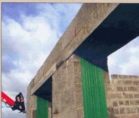
Underslab insulation in line with Perinsul block for continuous insulation (left); stainless steel cavity wall ties and inbuilt hoses for injecting full fill insulation (centre); and 200 mm cavity closers (right) are fitted to all openings in the cavity
