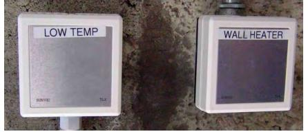
Over summer 2009, this frost thermostat *(improperly set at 17°C on installation)* energised the wall heater in a plant room of a new low-energy building, and wasted more electricity than the wind generator *(designed to offset the entire building's annual heating energy use)* created.
