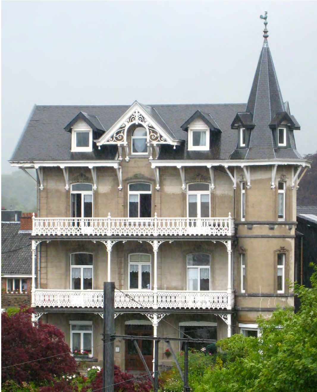
Figure 3. The characteristic features of traditional ‘greatcoat’ architecture, such as wide eaves and hood mouldings, may appear decorative, but their primary purpose is entirely practical: to stop rainwater penetrating weak points of the wall. ©Clive Murgatroyd.
