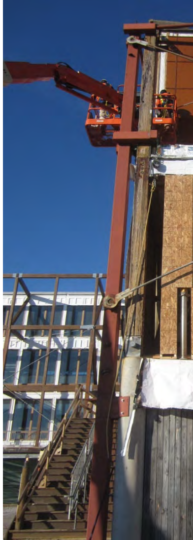
Figure 5. Engineered wood structural members expressed on the exterior envelope of the building. Photo: Wiss Janney Elstner, Inc.
