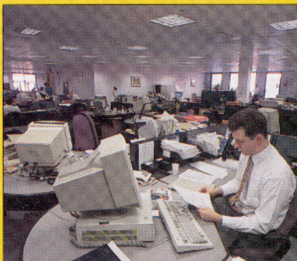
Spot tests by the PROBE team confirmed that the lighting provides 350-500 lux on the working plane. At 36 kWh/m 2 , the lighting energy consumption is low by typical 1980s standards.
