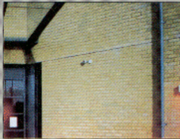
The external air temperature sensor exposed to the sun.
