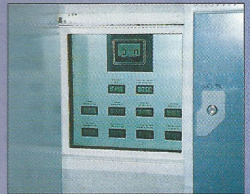
ABOVE: The bems summary display panel, intended to provide pupils with an insight into the building's performance, is not operating reliably.
