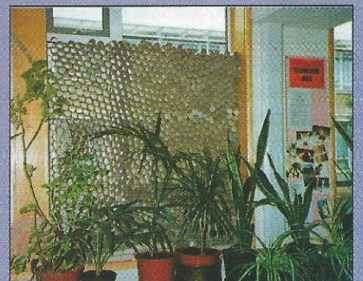
Do-it-yourself transparent insulation – stacked toilet rolls do the honours in the art studio. A patent beckons, surely...
