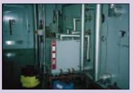
One of the rogue humidifiers which often runs in summer to replenish the moisture that is removed at the cooling coil.
