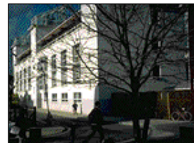
#18 POR The Portland Building
