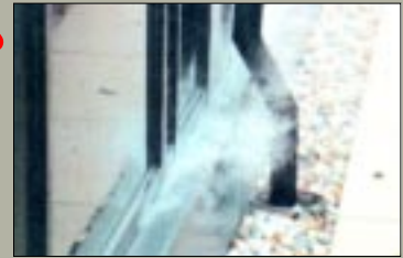
Gardner House: air leakage seriously affected fuel efficiency and comfort levels.
