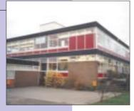
2. Lights on, blinds down – and wonky: a variation on a well-worn theme particular to school buildings. This is evidence that good façade detailing – inclusive of window design, solar shading, blinds and window opening mechanisms – must be very carefully integrated to optimise daylighting and ventilation control strategies.
