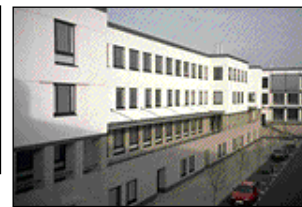
#14 FRY The Elizabeth Fry Building
