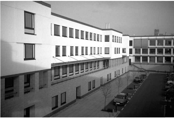
Figure 3 The Elizabeth Fry Building (left). Photo: Bill Bordass Note: FRY had the lowest heating energy consumption in Probe. It has lecture rooms on the ground floor, seminar rooms on the first floor, and largely staff offices above. Highly-insulated fabric and triple-glazed windows with mid-pane blinds minimize unwanted heat losses and gains and made perimeter heating unnecessary except in five corner rooms. Heating, ventilation and cooling is provided by blowing air through the hollow cores of the structural floor slabs. The ventilation plant operates during occupied periods, with heat recovery until embedded sensors in the floor slab reach 22°C. If slab falls below 21.5°C the air is also heated. Overnight, the fans operate to pre-cool the building if slab temperatures are above 23°C and it is at least 2°C cooler outside. Windows are openable if occupants wish. After monitoring and fine-tuning, this building achieved exceptionally high levels of occupant satisfaction for its office staff, together with low energy consumption.
