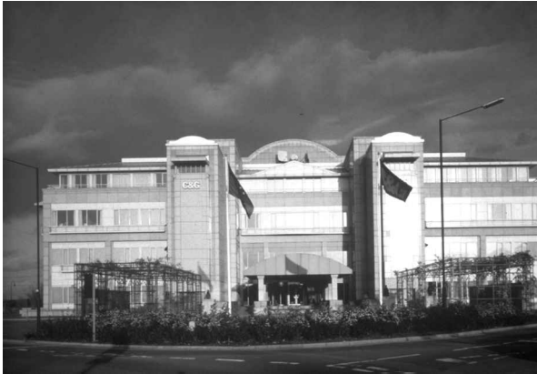
Figure 7 The Cheltenham and Gloucester Building Society's head office near Gloucester. Photo: Bill Bordass
