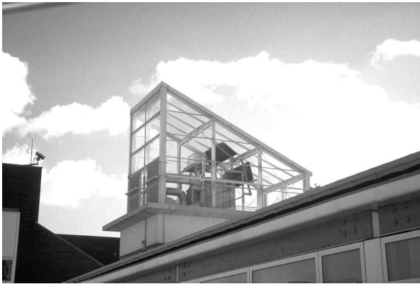
Figure 1 Turrets at the Portland Building. Photo: Bill Bordass Note: Five glazed turrets help to express POR's environmental control systems architecturally. They contain motorized windows which (with mechanical assistance where necessary) allow air to be exhausted, via the stair towers, from ceiling bulkheads running down the middle of the occupied floors below. Some turrets – like this one – also contain small solar panels for preheating. However, the gas-fired boilers in the plant rooms immediately below are not condensing.
