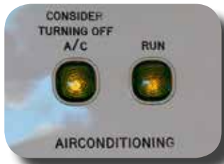
Figure 6: Wall-mounted natural ventilation indicator panel visible to all users.
