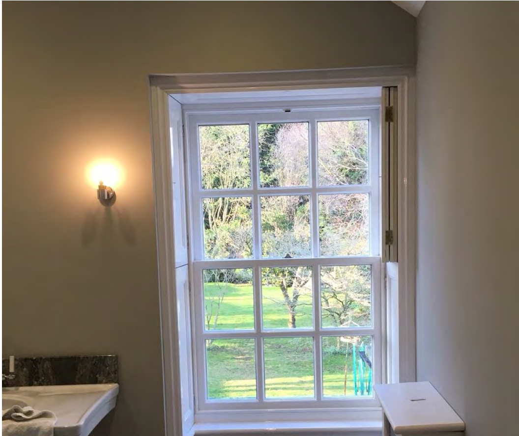
Figure 5.4: CS6's UPVC replica sashes and shutters in the Victorian bathroom with internal wall insulation
