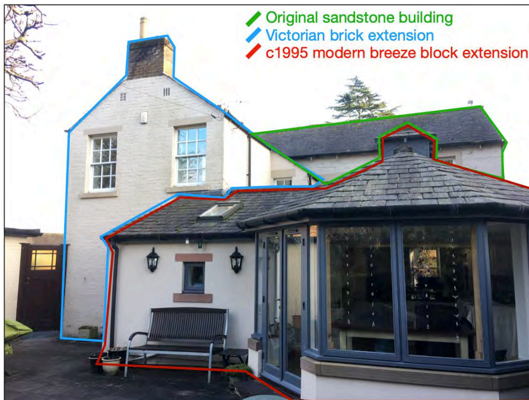
Figure 7.6: CS6, poor form factor with several complex elements
