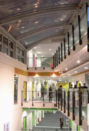
**Hackney Academy.** Extract air from the classrooms is drawn into circulation areas via colour-coded grilles and extracted at high level via motorised glazed fanlights beneath the inflated ETFE roof.
