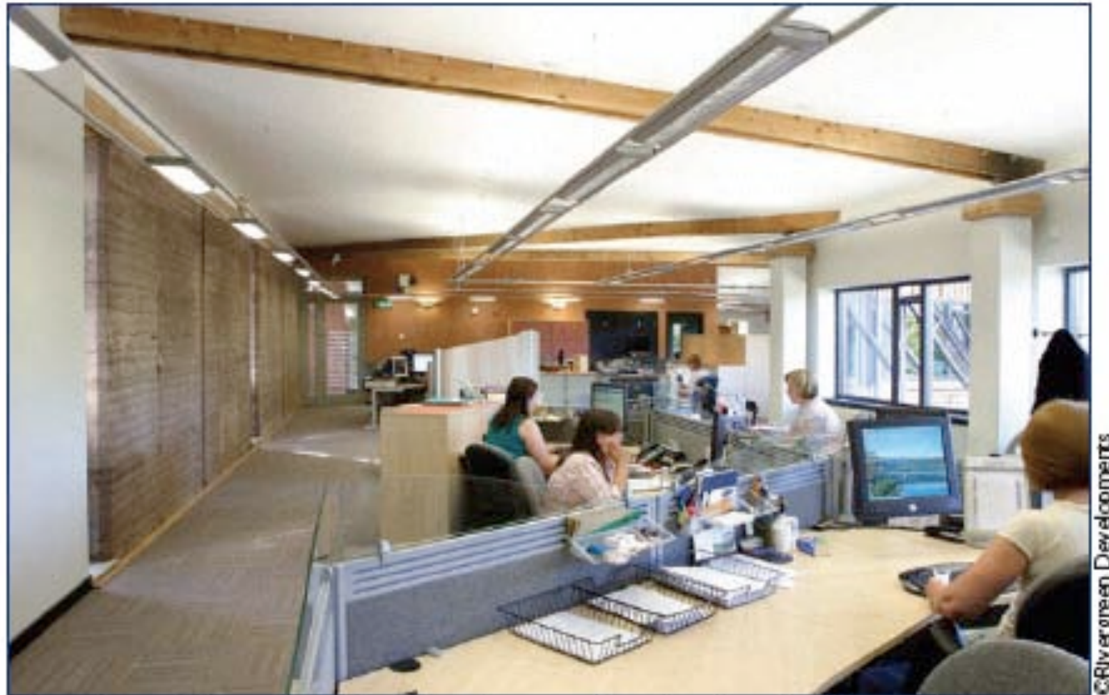
Above: A typical open-plan office. Note the rammed-earth wall to the left, openable windows and T5 dimmable fluorescents (controllable by hand-held controllers). The corridor zone has underfloor heating to accommodate future full-height partitioning.
