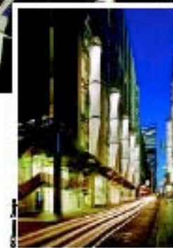
Above: The shower-coolers on the south side of the building supply evaporatively-cooled air to the shop area. They are claimed to reduce air supply temperatures by about 3°C. (After legwork was detected in the tanks, some parts of the system have been replaced.)
