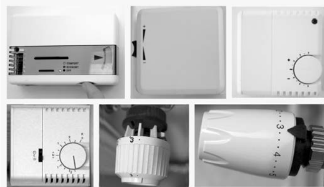
Fig. 1. Examples of typical room thermostats and thermostatic valves in Finnish offices.
