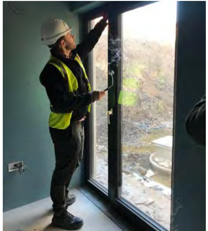
Illustration of one possible approach to identify source of leakage: smoke pen. (Source: Enhabit)
