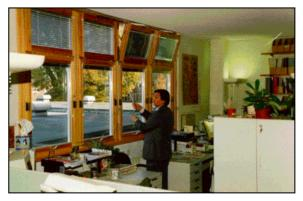
The windows in the design studio refurbishment at the Open University's Harold Wilson building were designed to avoid airconditioning and provide good user control. In spite of this there are still significant differences in occupant comfort between window and aisle seats [Reference 9]
