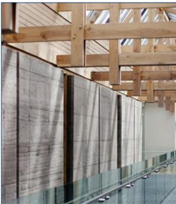
The Rivergreen Centre has a 6 m high, 500 mm thick rammed-earth wall inside the atrium. Being south-facing and subject to direct solar gain, the wall absorbs the sun's energy during the day and releases it at night and early morning to pre-heat the adjacent offices prior to occupation.
