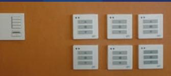
Locating user controls away from the devices they control – and not providing descriptive labels – invites problems. At Rivergreen this does not seem to be an issue yet as the building is otherwise user-friendly.
