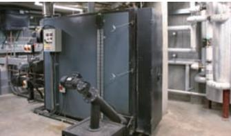
Experience at Rivergreen – and elsewhere – has shown that biomass boilers have difficulty operating intermittently as a conventional fossil-fuel boiler. Continuous running tends to be the outcome. The supplier is upgrading the boilers at Rivergreen to improve performance.
