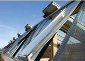
The atrium glazing vents are opened by the bms when a temperature setpoint is reached. User override controls are also provided on the atrium corridors so that occupants are able to deal with any discomfort themselves.
