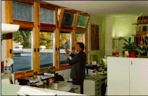
The windows in the design studio refurbishment at the Open University's Harold Wilson building were designed to avoid air-conditioning and provide good user control. In spite of this there are still significant differences in occupant comfort between window and aisle seats [Reference 9]
